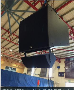
EV EVF - 2151D sub cabinet with EVU 2082 front fill ready to be flown into position
